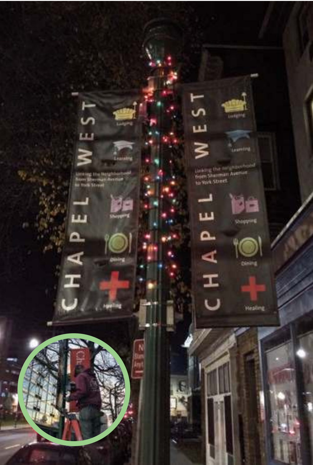
Colorful seasonal lights have been installed by DHL Electrical Services on 65 Chapel West district utility poles. More will be added next year as our budget allows.
