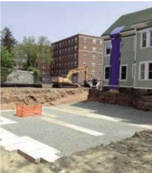
Newly poured foundation for the house awaiting its move
