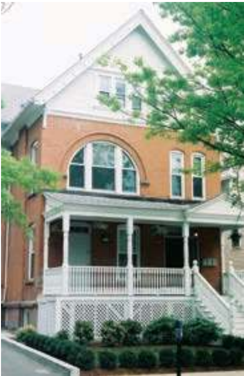
1195 Chapel St. with its brand new porch.
