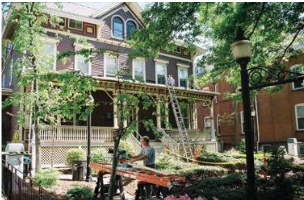
Renovations at AYA
