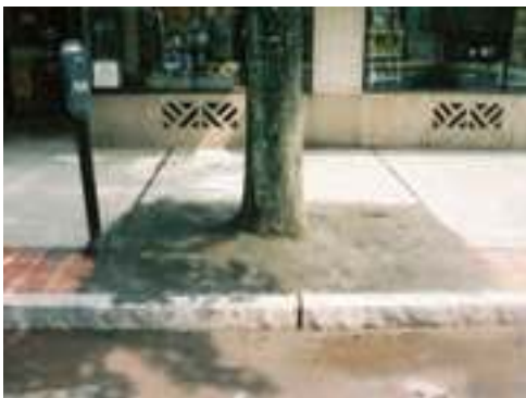
After: Poured concrete has replaced the bricks. Gravel around the trees allows for future growth.
